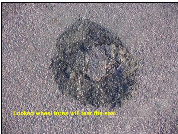
Locked wheel turns will tear the seal
