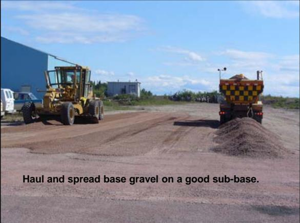
**Haul and spread base gravel on a good sub-base.**
